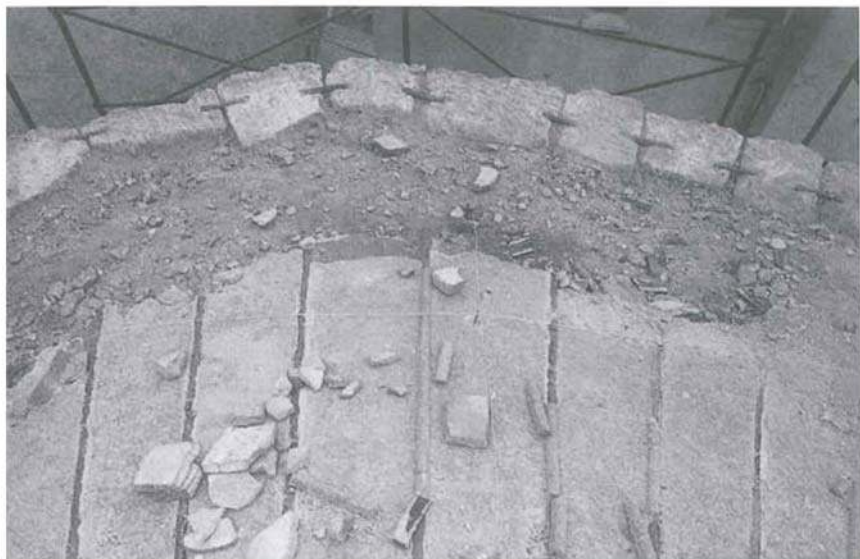
Figure 1. Istanbul, Zeyrek Camii, south church, green stone cornice blocks over the eastern wall (A. Neftçi, 1997).
